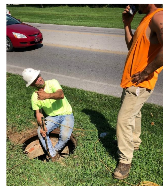
Bill Cornett, left, holding fiber optic cable end talks with Aaron Rice relaying information by radio. The two work for Triple D Communication, the company which is doing much of the installation for MetroNet.
