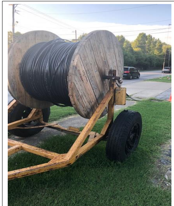
Fiber optic cable, about a mile away, being pulled underground. Underground internet cable is less likely to be interrupted by storms. These pictures taken on Clays Mill Road.
