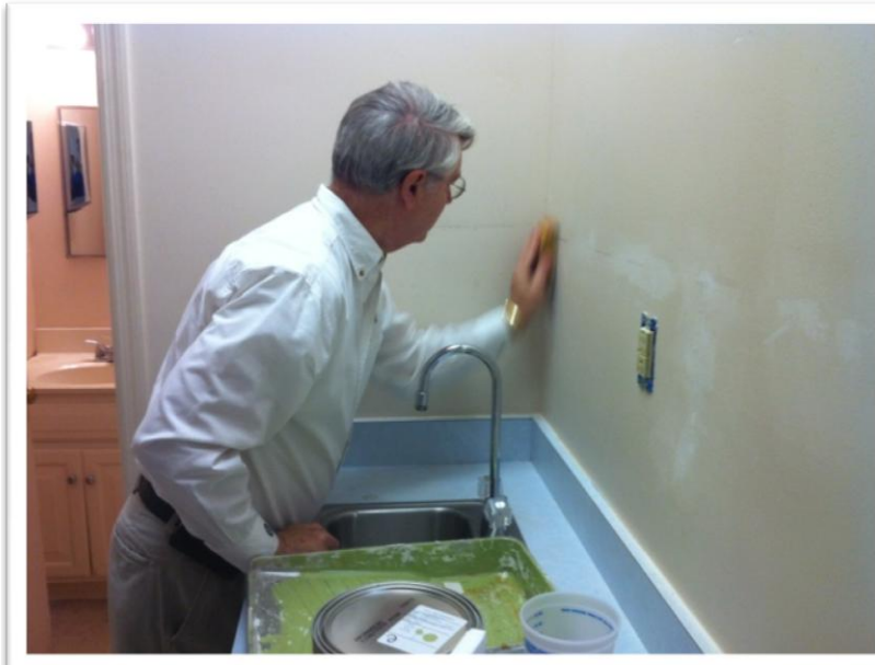
In preparation for painting, Larry Neuzel sands a wall where a shelf once was located
