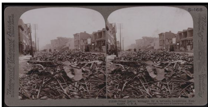
From 1913: Louisville suffers major damage from a tornado that struck Kentucky's largest city. Photo shows debris strewn throughout the street. Photo is titled, Great havoc wrought by a tornado, Louisville . Photo is on card mount. The stereo view was copyrighted by Underwood and Underwood. Location of damage in Louisville and photographer are unknown.
