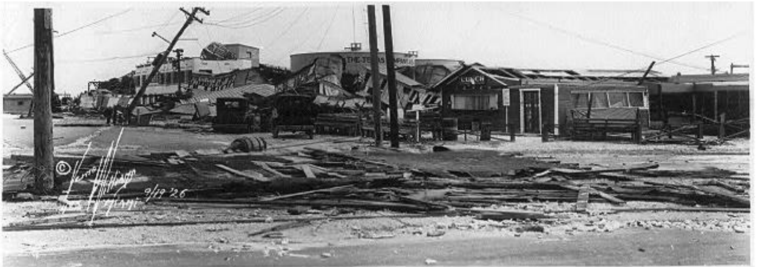
Oct. 9, 1926: Severe hurricane damage recorded in Miami, Fla.; from a photographic print. Photographer: Verne O. Mills of Miami.
