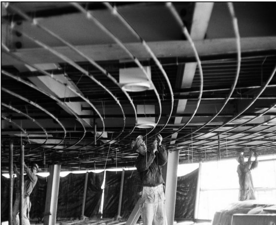
Construction workers building the Seattle Space Needle, in early January 1962
