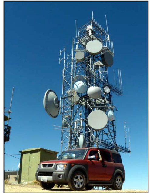
Communication tower shown in Sept. 2008 with dishes for microwave relay links on Frazier Peak in the San Emigdio Mountains, Ventura County, Calif. It serves the Mountain Communities of the Tejon Pass, and other entities. The dishes have radomes, plastic sheets covering their apertures, to keep moisture out.
